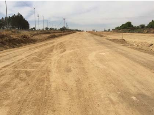
Roadbed KM 8+680 to KM 8+920
