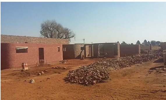
Boipatong Social Intergrated Facility :Early Childhood Development Centre
