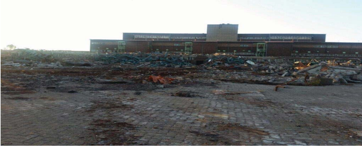
Old Natalspruit Hospital Demolishing
