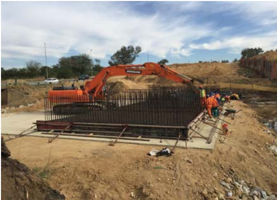
Culvert No. 5601 KM 9+180
