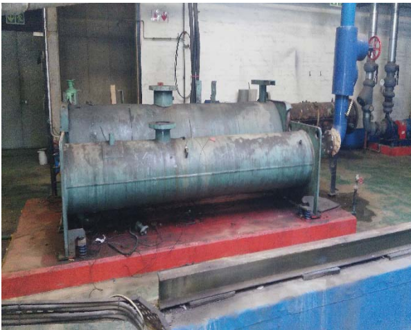
78 Fox building: Replacement of boilers & chillers
