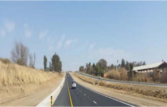
Final road mark
