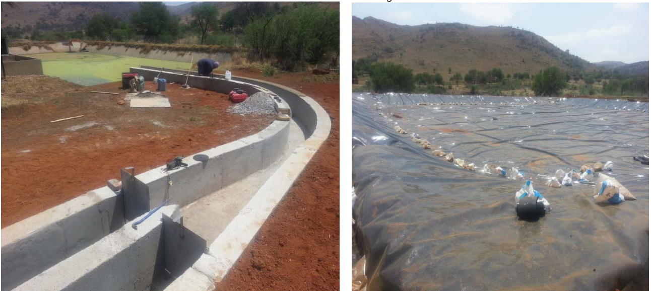
The membrane laid in the Oxidation Tank at Suikerbosrand Nature Reserve during construction
