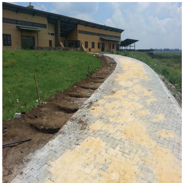
The bedding and kerbing completed, and then laying of paving blocks
