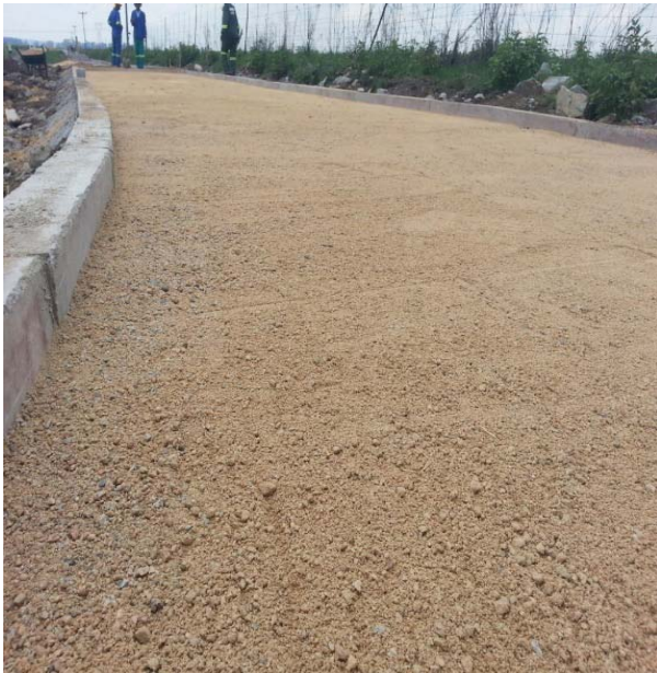
Construction of Road at Marievale Nature Reserve blocks
