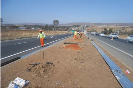
Installation of median guardrails
